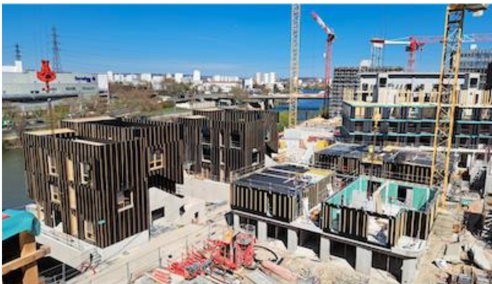
Travaux lot PB10 ©Thomas Charmasson Gipen
